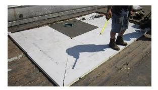
Oftentimes, building owners will agree to have a tapered insulation system installed only to have it value engineered at some point during the process, reducing the roof system's efficiency and increasing the potential of creating problems down the road.
