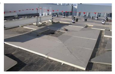
not provide adequate slope. A properly designed tapered roof insulation system not only provides the necessary R-value and the support for the roof system, but it helps extend the life of the roof system because it provides the required drainage.<sup>2</sup>
